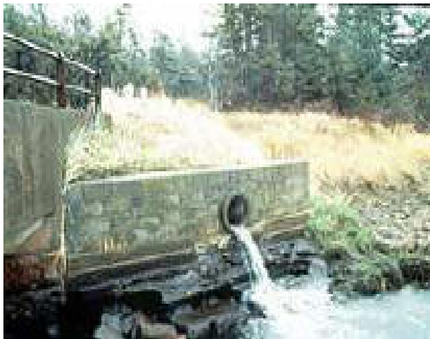
Drainage outfall
