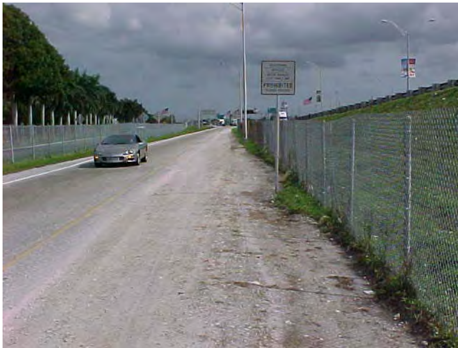
Exhibit 8. Gravel shoulder along westbound Ludlam Road exit ramp
