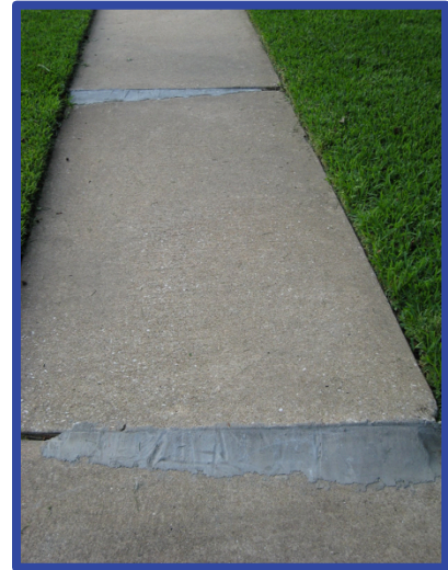
Figure 4 - Patching and Ramping
