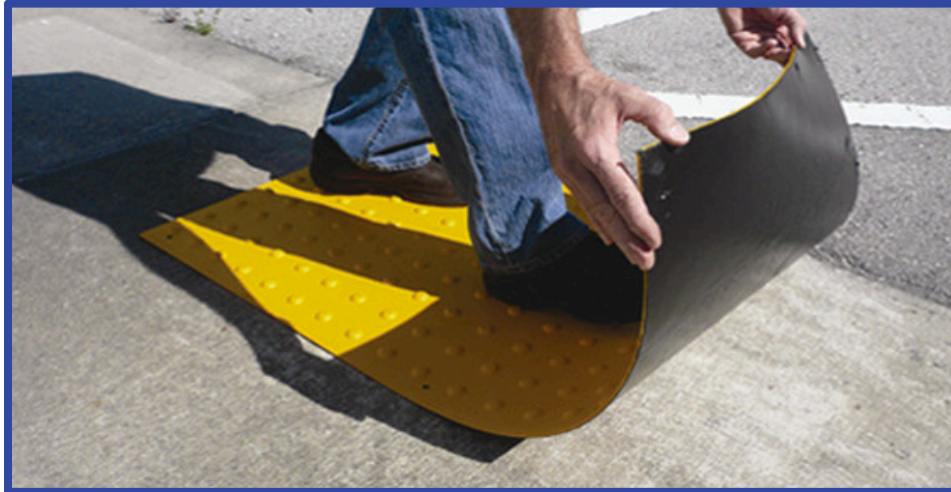
Figure 5 - Detectable Warning Installation
