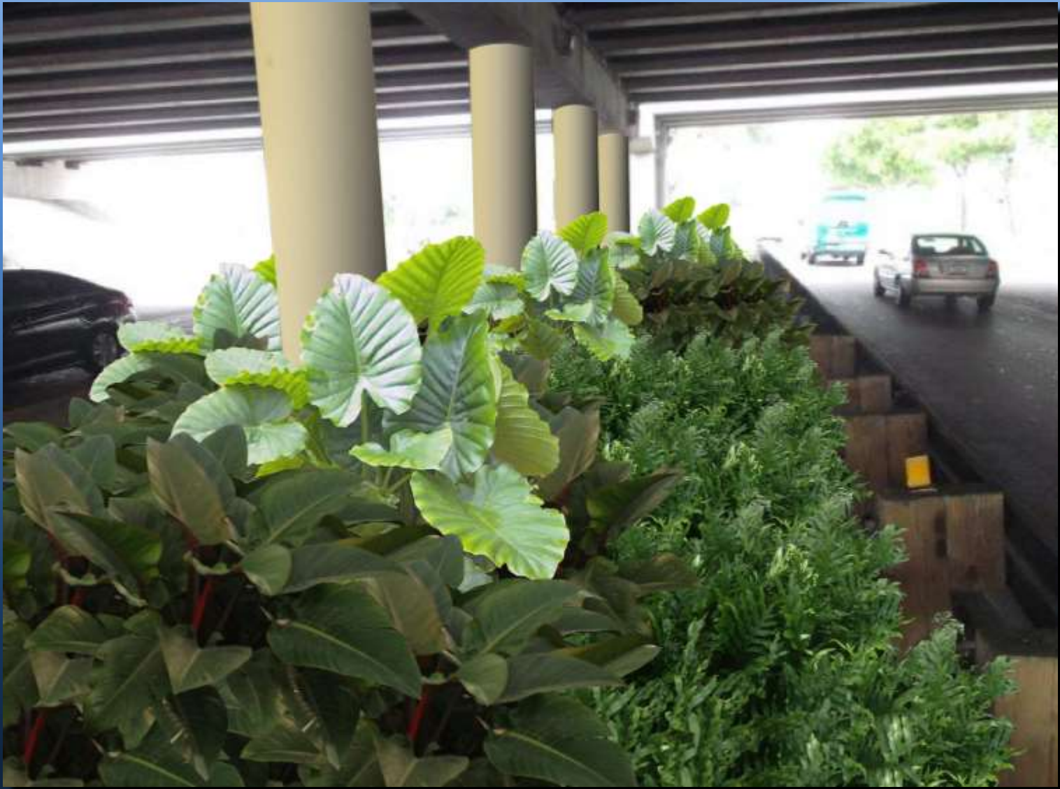
UNDERPASS WITH LANDSCAPING AND PAINTED CONCRETE COLUMNS
