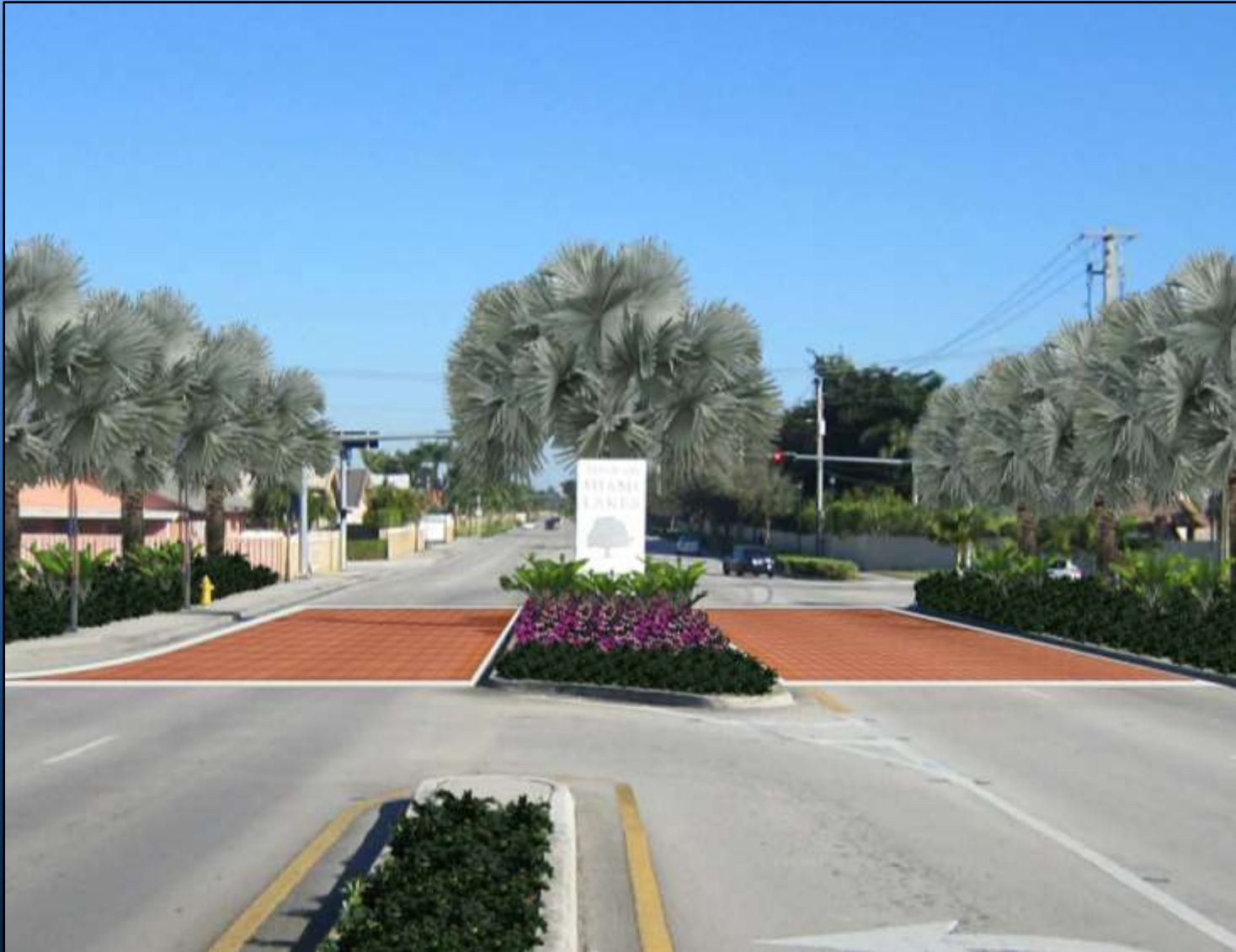
GATEWAY WITH BISMARCK PALMS, GROUNDCOVERS & SPECIALTY PAVING
