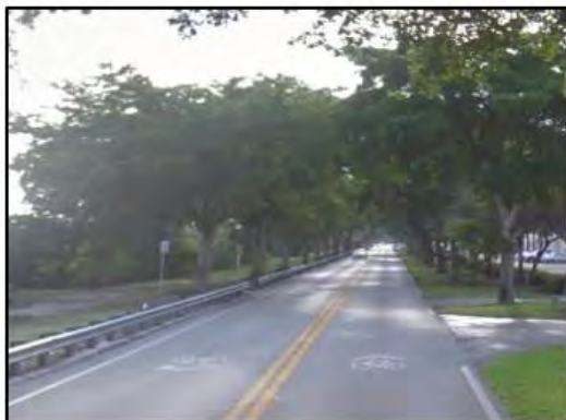
NW 77 th Court (Southwest bound) - Commercial
