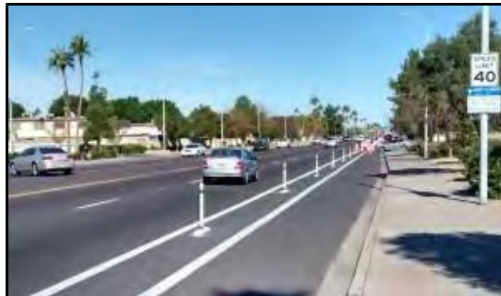
Figure 11: Barrier Separated Bike Lane – Delineators/Flexposts
