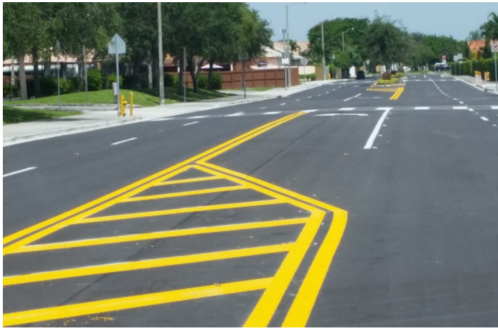
WEST LAKES A PH-I—DRAINAGE IMPROVEMENTS
