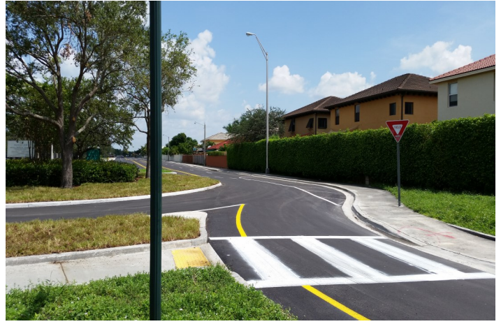
WEST LAKES A PH-I—DRAINAGE IMPROVEMENTS
