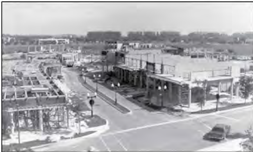
Early construction views of the Main Street shopping area
