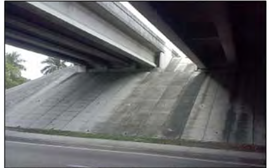
Existing embankment condition under Palmetto Expressway at NW 154th Street
