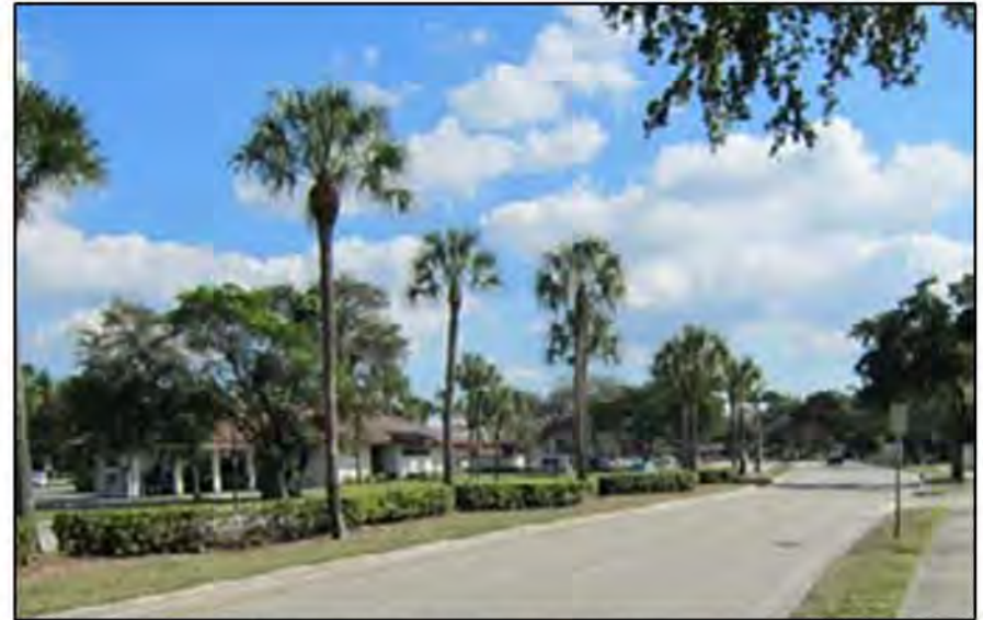
Existing condition along Miami Lakes Drive (Major Roadway Type 1)
