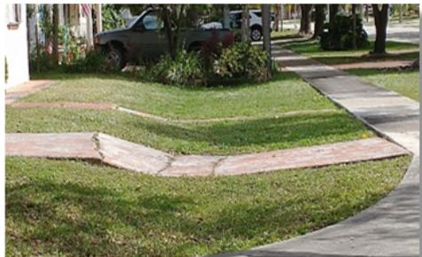
Liquefaction is a known phenomenon when energy is introduced into saturated soils. Soil substantially loses strength and stiffness in response to an applied stress such as shaking during an earthquake or other sudden change in stress condition, in which material that is ordinarily a solid behaves like a liquid.
